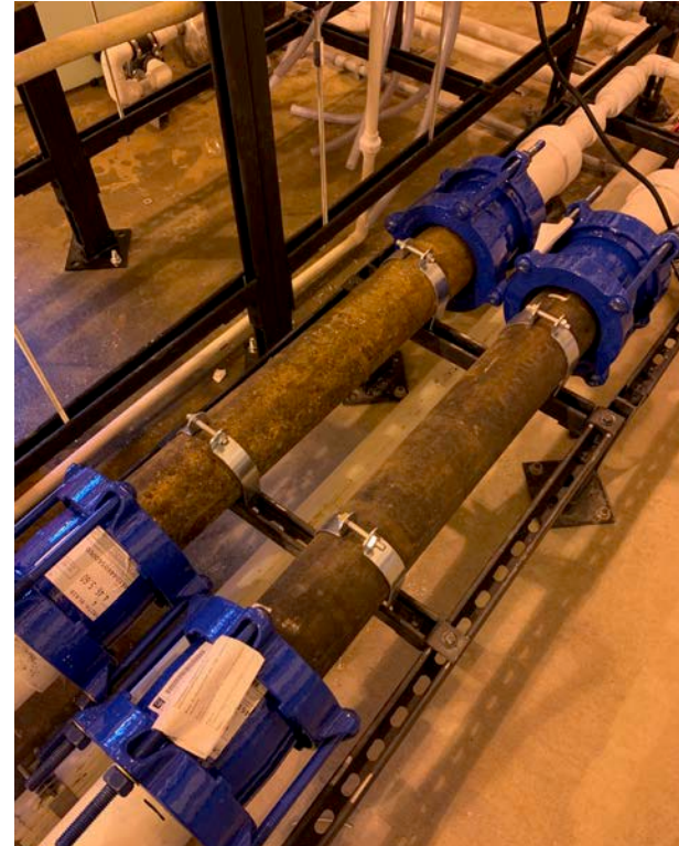
Harvested Cast Iron and New Ductile Iron Mains
